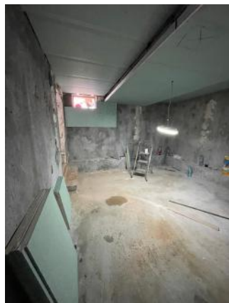
The basement renovation continues. It is coming together!
